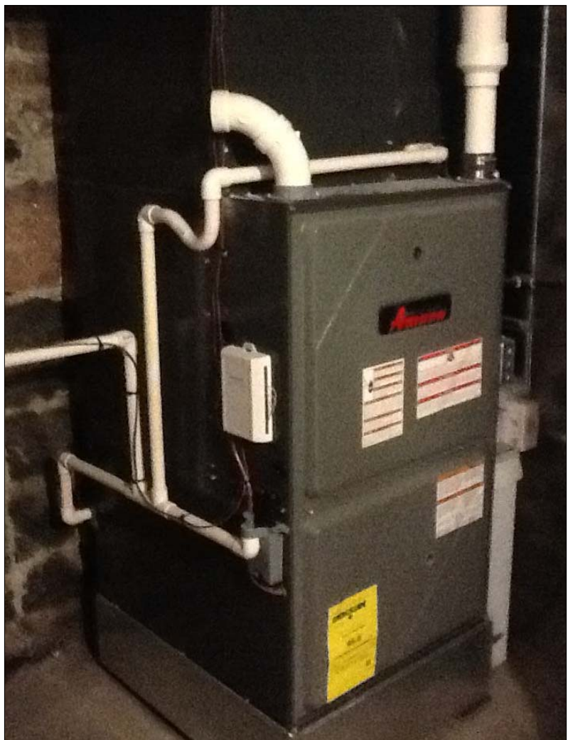
New heating and AC.
