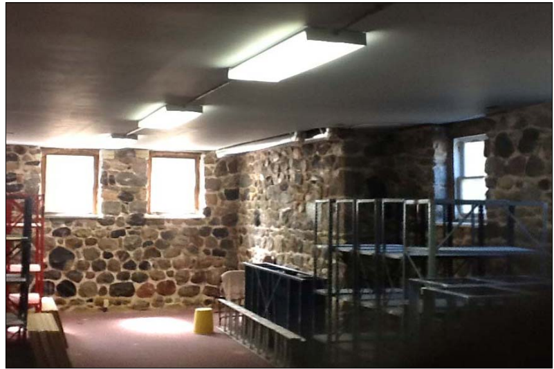
Let there be light - new basement lighting.
