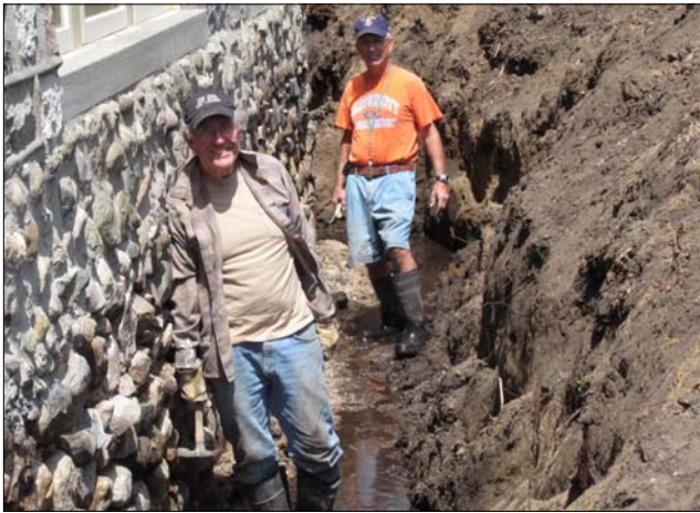
Ross and Dan in the trenches.
