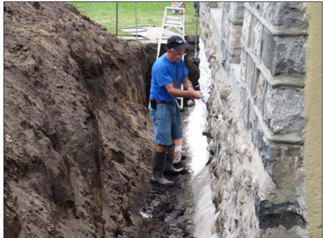
Applying a water barrier.
