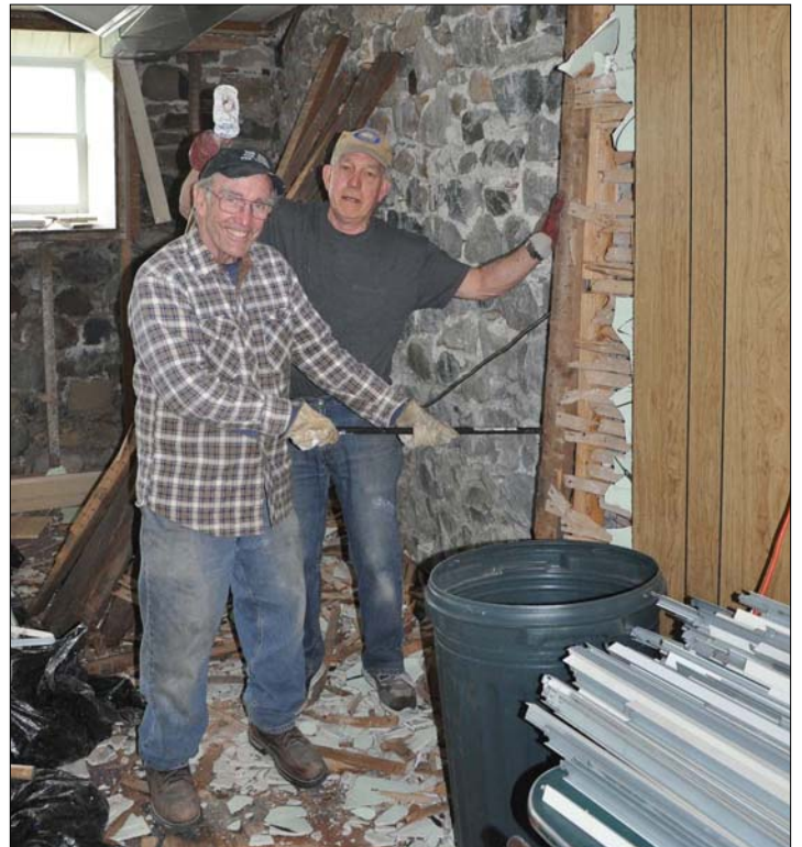
Ross Graham & Howard Richter removing plaster and lathe .
